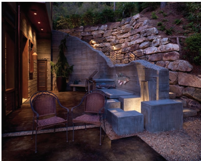
Step lights provide safety on the stairway while an underwater light accents the water feature.
